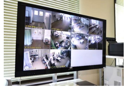
Video surveillance system is monitoring facilities.
